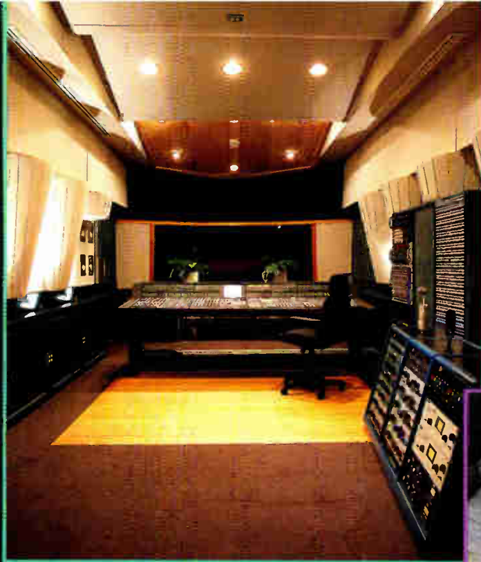
A&M renovated Studio C last year, implementing acoustician Vincent Van Haaff's innovative designs for 5.1-channel mixing. The studio houses a 96-fader Euphonix CS3000M, Sony PCM 3348 tape machines and a large complement of vintage outboard gear. Main surround monitoring is a custom dual-concentric, DTS-ready system consisting of PAS/TAD components.
