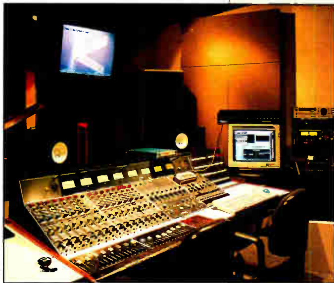
Control room C at Post Modern Sound, Vancouver, BC: online/offline
