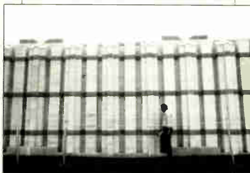
Rear diffusor wall at Starplex Amphitheatre
