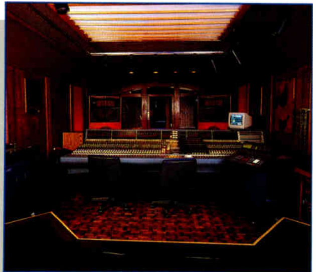
CONTROL ROOM II
