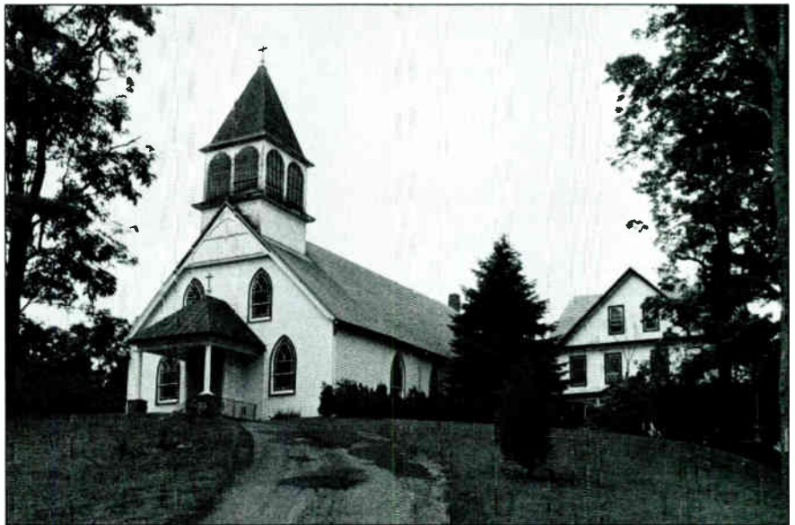
Exterior of the 100-year-old facility.
