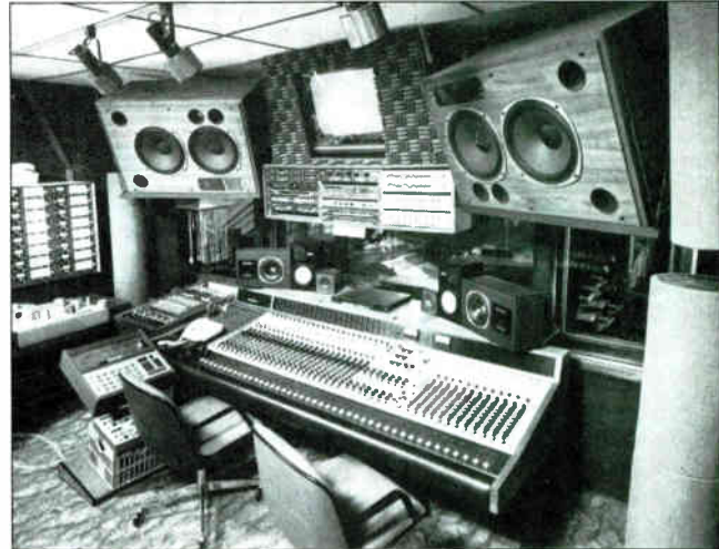
Millbrook Sound Studio (in Millbrook, NY) became the first studio in the state to install Tannoy's 15-inch FSM rock monitors powered by Tannoy's SR840 hi-current MOS-FET amp. It was installed by Richard Rose of Hot House Productions of Highland, NY. Recorders in the studio include an Ampex MM1200, Otari MTR-10 and MTR-12. The console pictured is a NEOTEK Series III.
