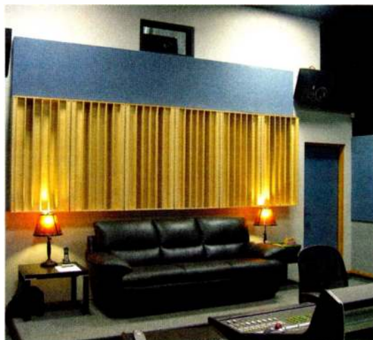
Rear view of mix room with fabric-covered absorber panel between QRD diffusers and projector portal
