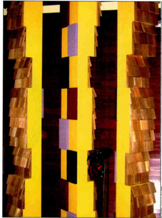
Acoustician Terry Hazelrig used three rotating vertical panels to surround Fur Seal's drum area.
