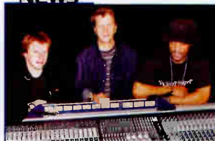
A.C. Lighting (Buckinghamshire, UK) installed a 40-channel Soundcraft MH4 in London's Hackney Empire. Pictured from left: engineer Paul Gavin, tech manager Brian Wren and chief tech Othman Read
