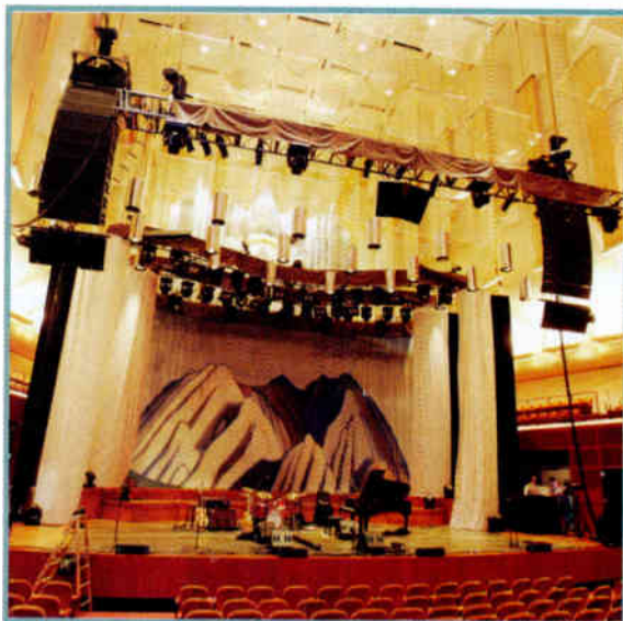
FOH engineer Dave Lawler uses a wireless tablet controller to test the Meyer Milo line array, as photographed at San Francisco's Davies Symphony Hall
