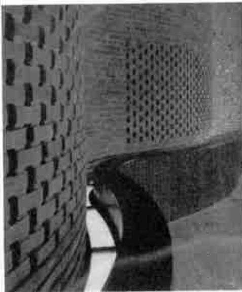
Fig. 7. Detail of the Chapel wall. No two curves are of the same radius, a design employed to avoid standing waves. Openings in the brickwork are a part of the acoustic treatment. They are used also for ventilation
