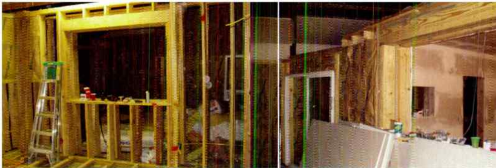
Room within a room construction: Sound Logic studios being built inside an old barn in the back yard. The photo at left shows the far wall to the control room being constructed. The middle photo shows the double wall design between the control and the tracking room. The photo at right shows the future control room, complete with two layers of sheetrock on each wall for solid soundproofing.
