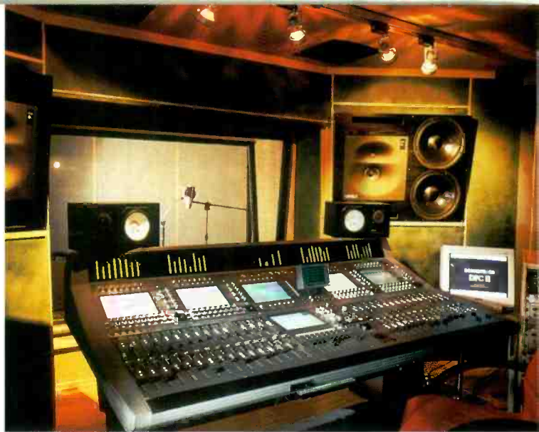
▲ Germany-UK: Paramusic, a recording facility based in Bensheim, Germany, has installed a 64-fader Soundtracs DPC-II console for owners and producers Roberto Rosan and Heiko Schmidt to ply their trade in hits with the likes of Sweetbox and Fuzion. A further DPC-II has been installed in Berlin's Sound 'n Picture film and TV post facility. The 48-fader console is part of a major refit adding a 24-track Augan workstation and incorporating surround working. Recent projects include Der Havelkaiser and various Disney productions. Meanwhile White Lightning Limited, owners of prestigious London post houses The Bridge , Silk Sound and Space have bought seven Soundtracs DPC-II digital desks as a part of the largest single refit project in the capital in recent years. Paramusic, Germany. Tel: +49 62 51 2535. Sound 'n Picture, Germany. Tel: +49 30 628 9280. Soundtracs, UK. Tel: +44 208 388 5000.
