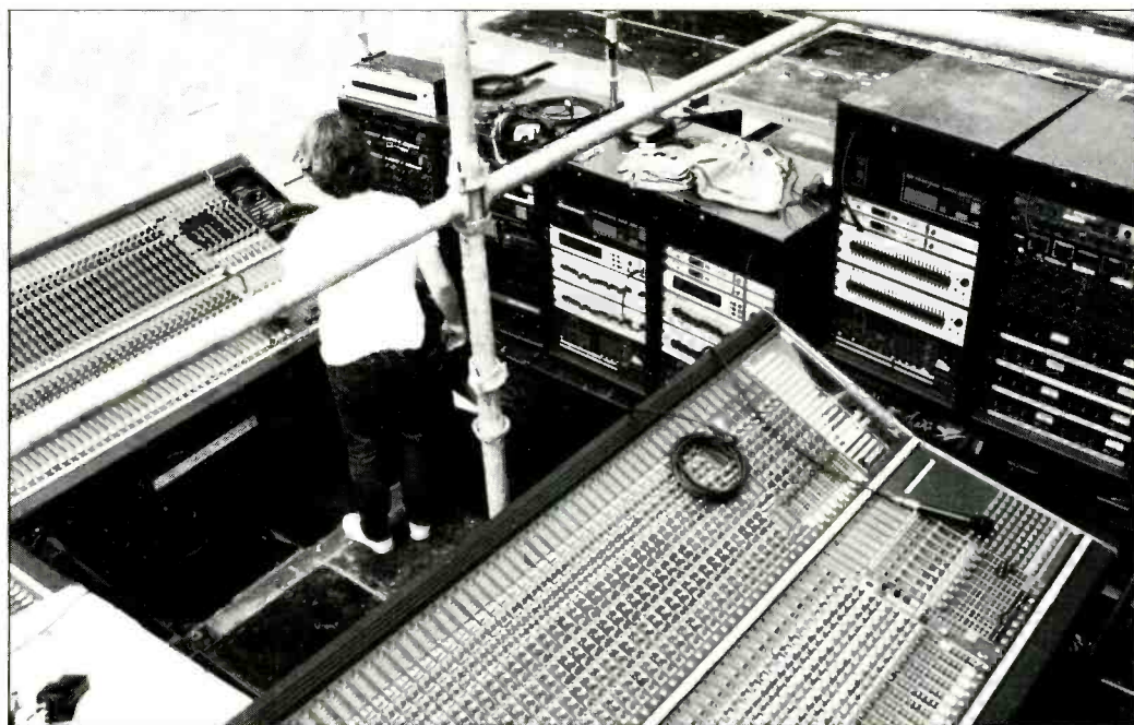
Front-of-house mixing position
