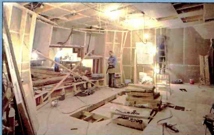
Control room under construction
