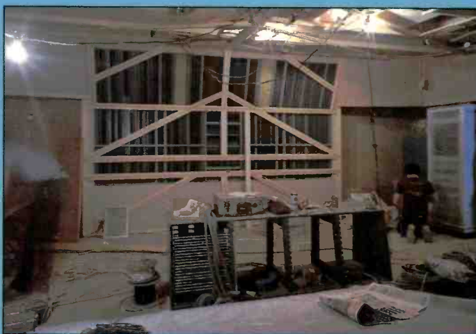
RPG diffusers at rear of control room
