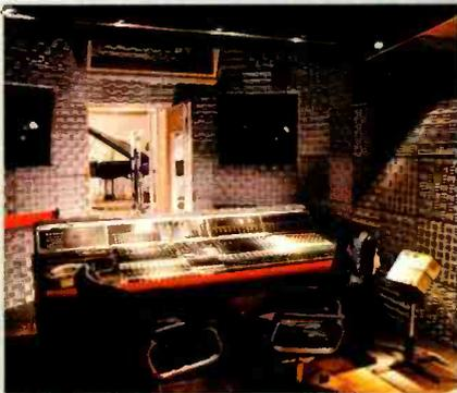
modular sound absorbers give a cost effective, flexible solution to acoustic problems. . .
