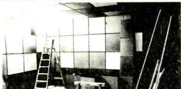
Installation of Sound Absorbers, Scripture Union, London
