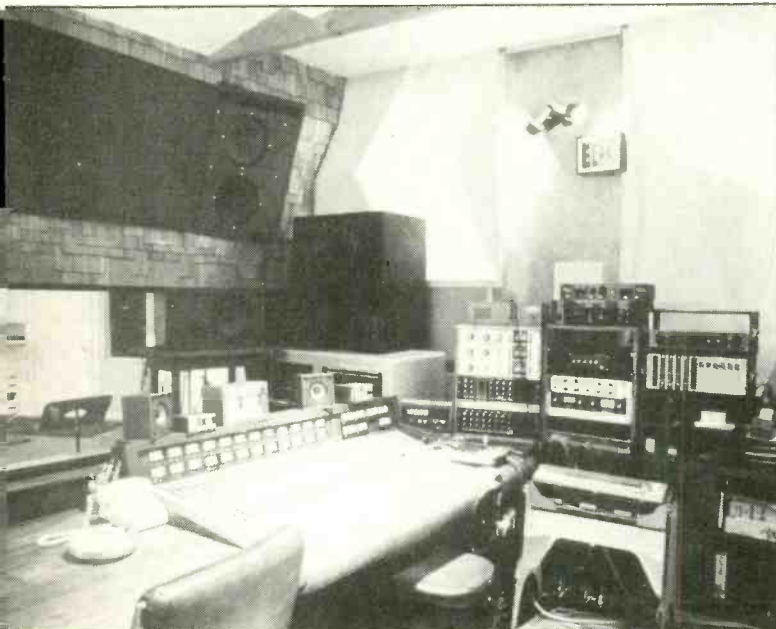
Above: Control room of Studio C. Right: Studio D nearing completion.
