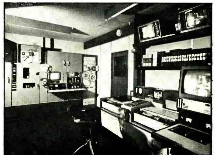
Top left: General view of control room, including audio and vision mixing equipment. Below left: Master video tape recorders. Rank Cintel 9000s. Below: Telecine area including Sony and Philips video cassette equipment and 35 mm flying spot scanner.
