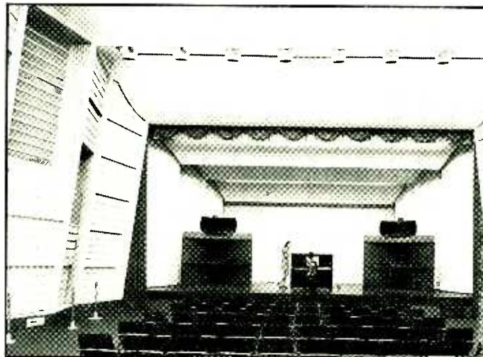
Victor's experimental studio in Yamato. The movable louvres, partly open, are visible on the left wall. Two of the four Mora playback loudspeakers can be seen on the stage
