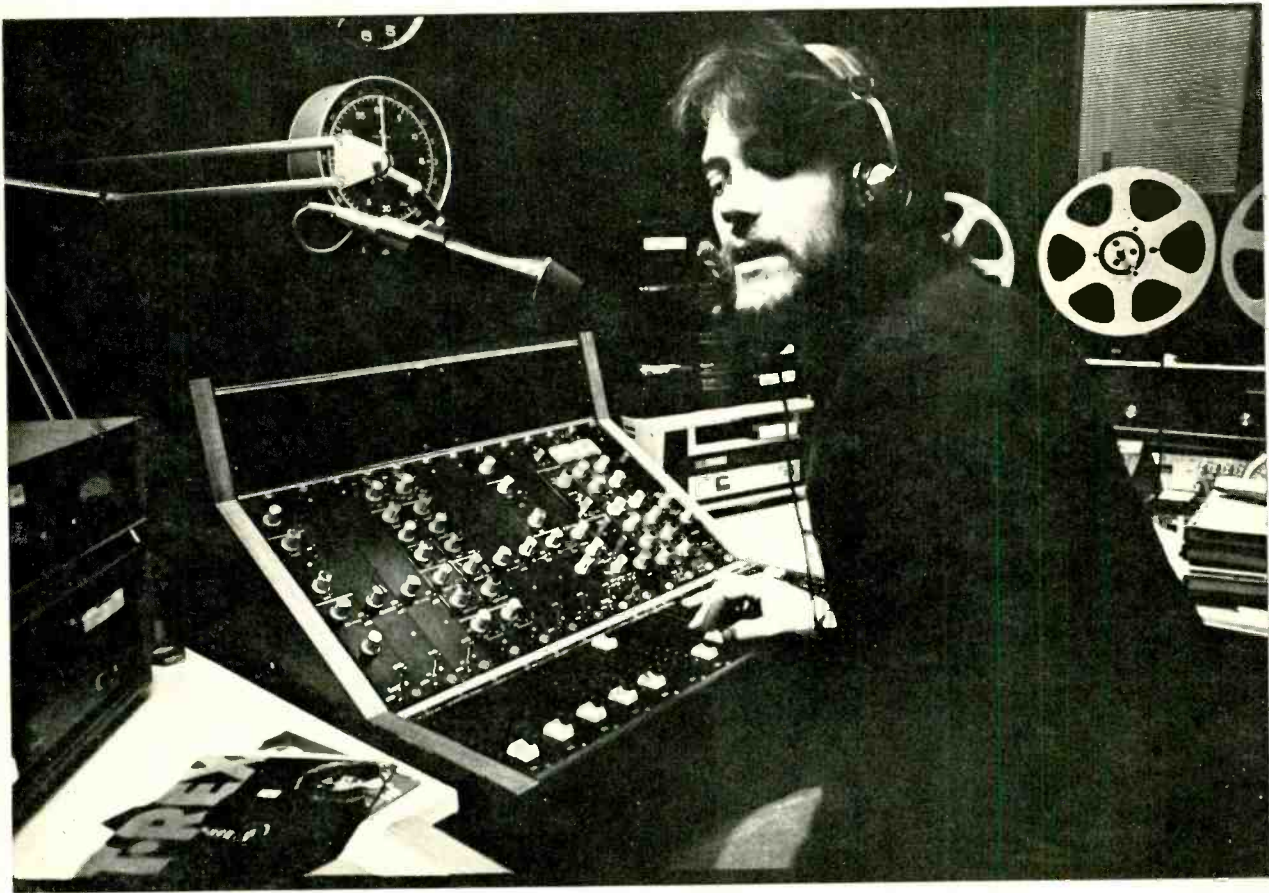
Mixer installed in the studios of Molinare Sound Services—10 Stratford Place, London, 01-529 0761
