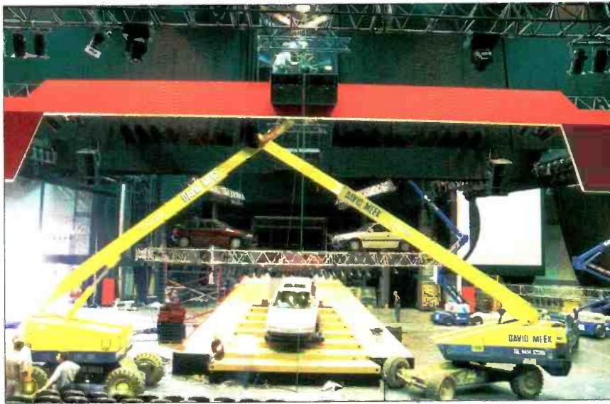
The speakers were flown at 22 motor hoist positions around the hall's 43 feet high ceiling, which comprises a network of steel grids with access for the riggers.
