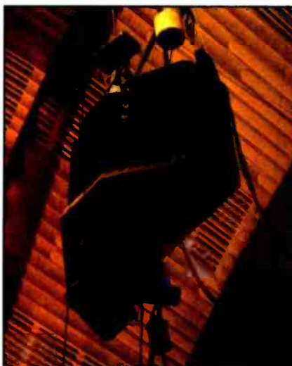
Photo 1. The center overhead speaker array included three of Apogee's 3x3 full-range enclosures, and three Apogee AE-5s, for down-thru coverage.
