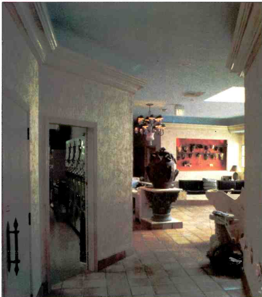
This hallway leads into the central machine room, located in the middle of the facility.
