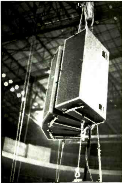
Figure 6. Custom compact metal hanging frames are used on the top and bottom of each speaker array.
