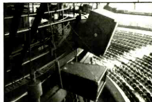
Figure 3. The second or outer catwalk supports the Spectra Sonics model 3000 cabinets. EAR horns and the AR microphone arrays. The circular unit shown lower left is for low-frequency pickup, while the cylindrical device next to it is tuned for midrange pickup.
