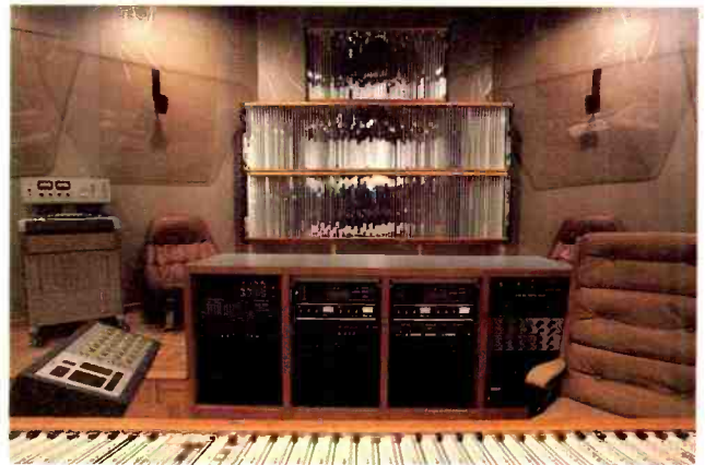
Rear wall showing diffusion/reflection
