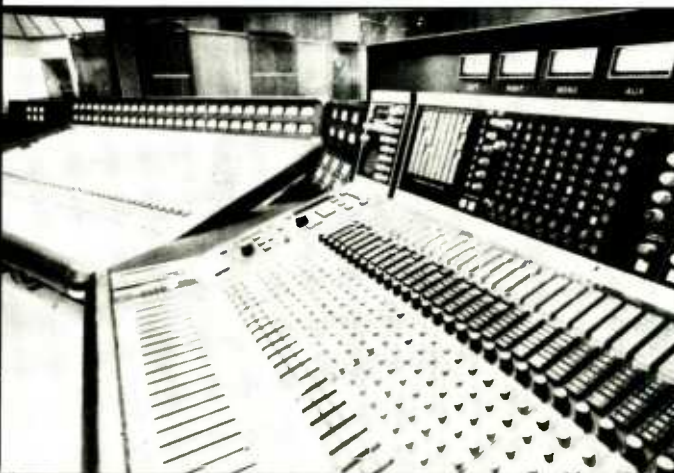
View across the sub-mixer to the control-room's main 40-input/32-output Solid State Logic SL 4000E automation-ready console, equipped with compressor-limiters on each channel.
