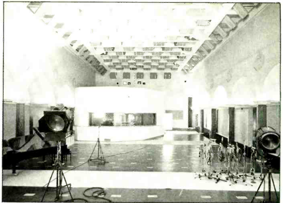
View from performance stage area along the length of the studio recording area to the corner control room. Clearly visible is the acoustic treatment applied to the unusually high and ornate ceiling. The treatment consists of V-shaped slabs of Rockwool "Rockfon" insulation suspended on cotton belts to save the cost of construction a supporting frame.
