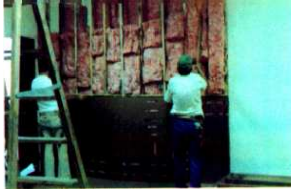
... bass trap under construction —
