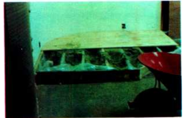
... ballasted drum booth base under construction —
