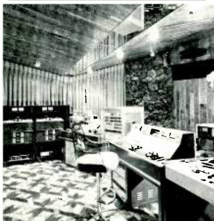
Photo of Kendun Recorders' mastering room depicts: (1) Angle between monitor (upper right) and stone wall; (2) Recessed tape machines for copies (master reproducer is adjacent to console); (3) Trap entrance behind curtain; (4) Compression ceiling.
