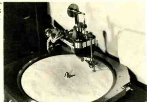
Léon Scott de Martinville's phonautograph, left, antedated Edison's phonograph by a generation. It could record but not reproduce sound. At right, Edison's own telegraph repeater. A recorder embossed a paper disc with the Morse code so that a reproducer (shown here) could later transmit the message. It was Edison's work on the telegraph repeater that led to his original phonograph, shown at center.
