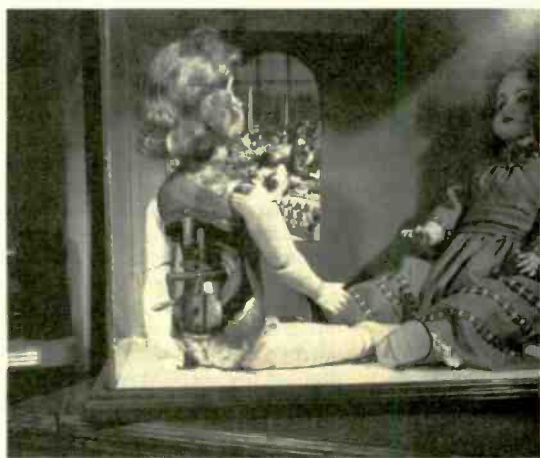
Talking dolls were the first consumer products to embody Edison's phonograph—and, later, Emile Berliner's flat-disc gramophone. The Edison doll, shown in its display case at the National Historic Site, used a hand crank as motive power. (Note the photo of the doll assembly line in the background.) Motive power for the phonograph at upper right was its water wheel at the far end, which was driven from a tap via a hose. This is the type of unit sent by Edison to pianist Josef Hofmann in 1890, referred to in "Notes to Future Scholars" at the end of "Recordings Before Edison" in this issue. The variety of recording and reproducing horns that Edison experimented with is almost endless—one recording horn measured 125 feet. Those at right are only part of the West Orange Historic Site collection.
