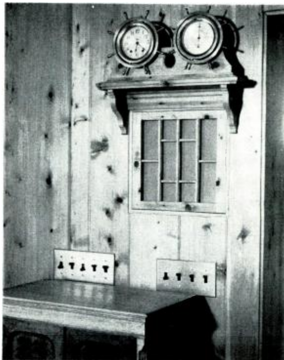
Fig. 9. Volume level of separate speaker located in bedroom can be regulated from bedside control box.
