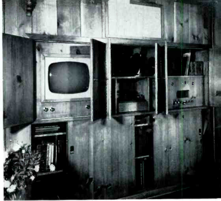
Building a system in a wall makes it neat and unobtrusive. When the doors above are closed, only the speaker grille shows.
