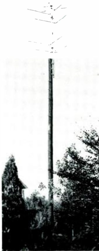
Fig. 7. Atop a 45-ft. pole are two individually rotatable antennas.
