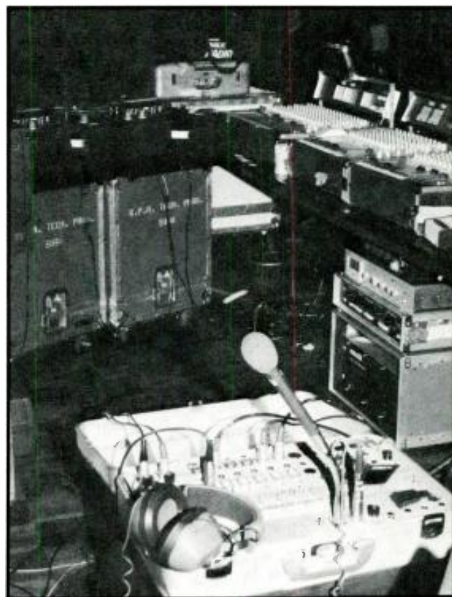
Figure 5. Director's position and mix area with IFB control panel in foreground.
