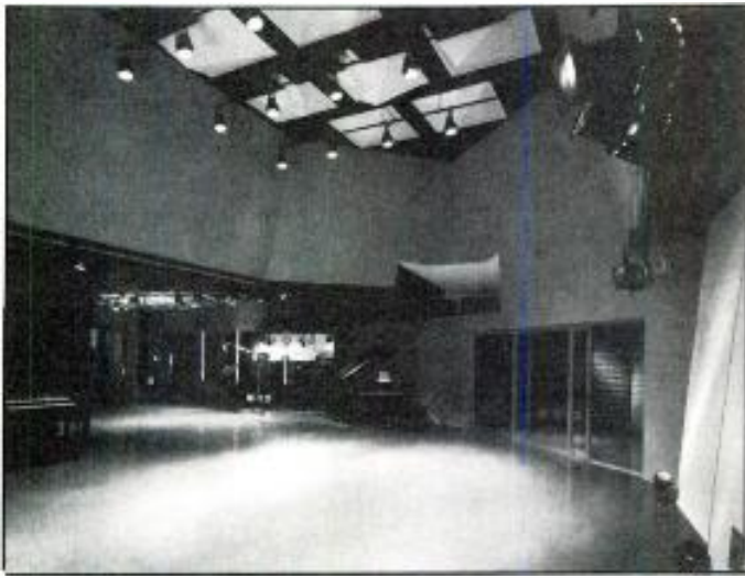
Figure 3. Studio A—live area. Note the diffusive and absorptive elements on the ceiling.
