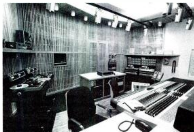
Figure 3. View toward rear of control room showing "tunable" screen wall.
