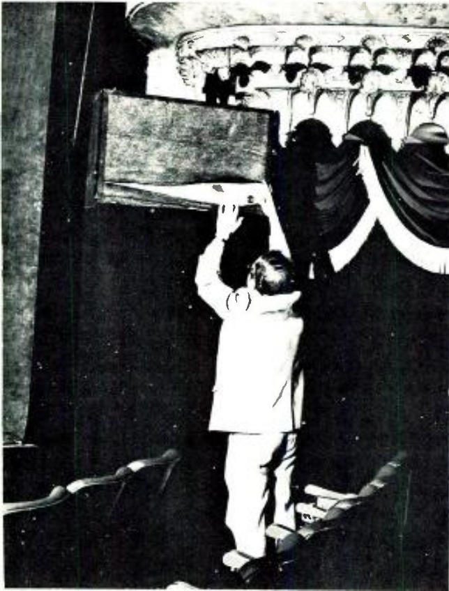
Figure 2. Two more Sentry IIs deliver all the sound from the stage performers. They are installed just a few feet from the proscenium, one on each side.
