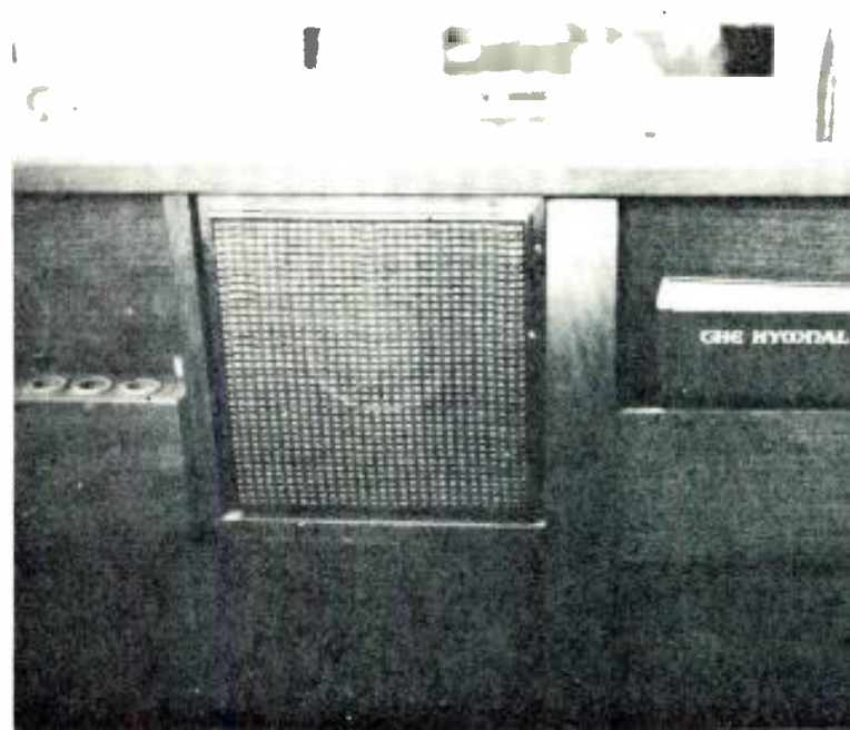
Figure 6. The pews on the balcony showing the individual speaker enclosures.
