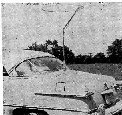
Fig. 8. Alford loop FM antenna on car.
