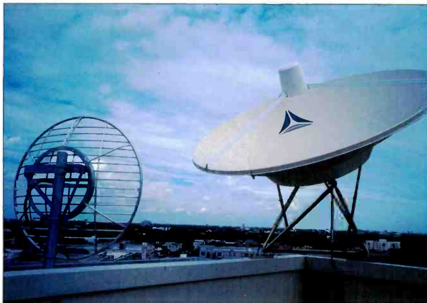
Since moving to the tower, classical station WTMI has improved its audio quality by replacing telephone program links with a microwave relay dish (left) and a satellite link to the Mutual Broadcasting Company's Metropolitan Opera feed (right).
