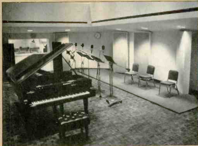
Fig. 5—WFMT Studio One. Note the adjustable absorber panels. The panels are rotated to vary the absorption-vs.-frequency curve. Additional panels, full studio height, can be placed as needed, on barely visible runners. The soffit shown spans most of two walls and houses support beams and the ventilation muffler system.
