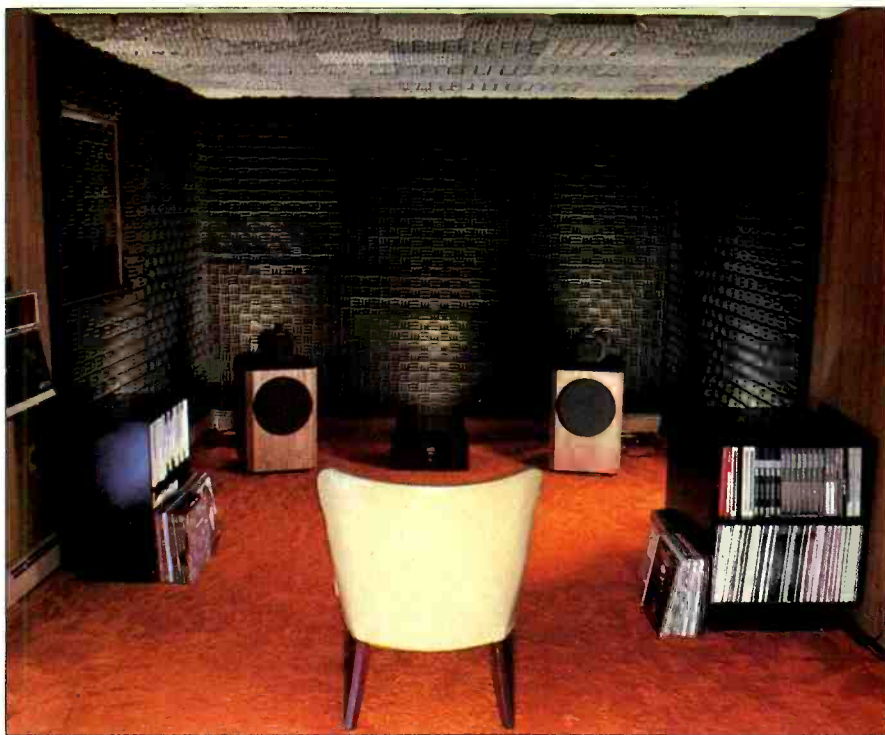
Bert Whyte's listening room, in which sound-absorbing Sonex was used in an LEDE installation.
