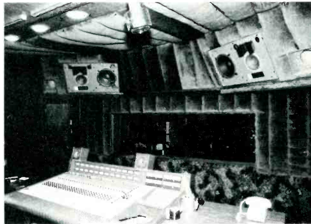
Fig. 9 — The dead end of the control room built by Chips Davis at Las Vegas Recording.
