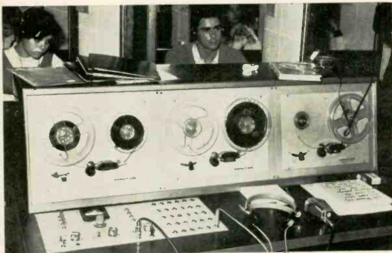
(Left), The control panel and master program source of the original language laboratory at The George Washington University which was one of the earliest in the country. (Right), One of the student booths employed in the original installation.
