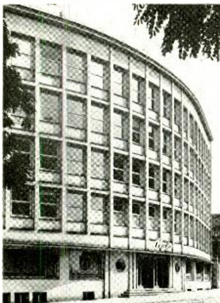
Main office and factory building of Metz in Fuerth
