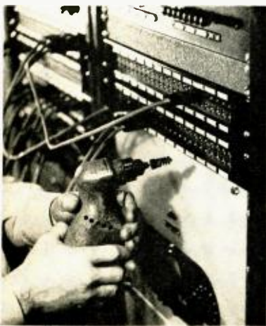
Fig. 1. Clean jack barrels with a brush chucked in a pistol-grip drill.
