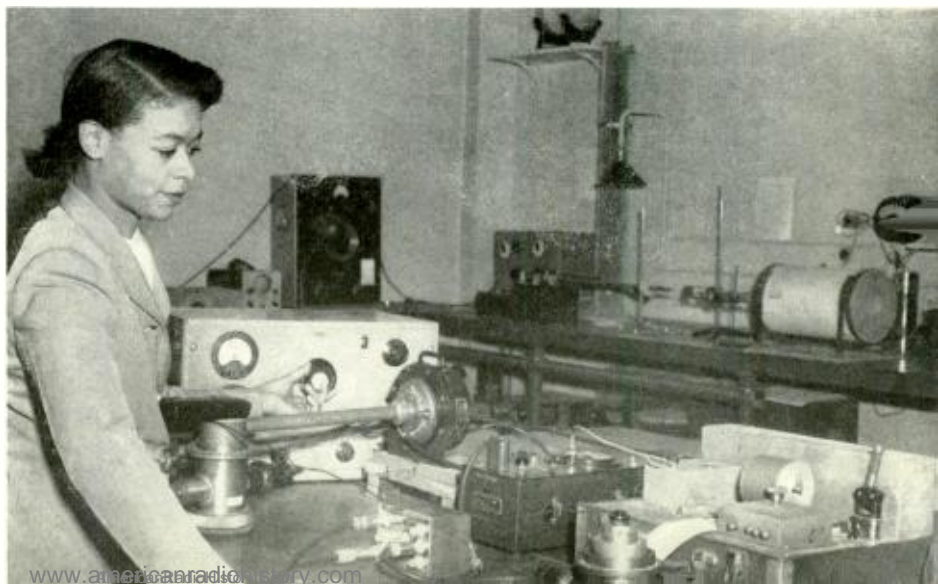
Fig. 1. Laboratory assembly of apparatus used for determining hearing aid gain by a cavity pressure method. Essential items include (left to right) driver oscillator, the source cavity and preamplifier source tube, loudspeaker element, electronic amplifier-voltmeter, and in right foreground, the "artificial ear" and its preamplifier, on which the hearing aid receiver is mounted. The power level recorder (right) is used here for automatic recording of data. The sound pressure level in either the source cavity or "artificial ear" can be recorded by switching the output of one or the other of the preamplifiers into the amplifier and recorder input.
