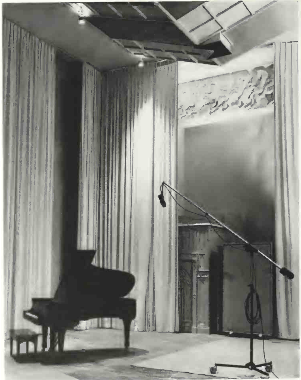
A portion of the main sound studio at Fulton Recording Company, showing the 24-foot high curtains on ceiling tracks which permit variation of acoustical treatment. Studio measures 50 by 35 by 24 feet, closely approaching the theoretically ideal acoustical proportions of 5—3—2.
