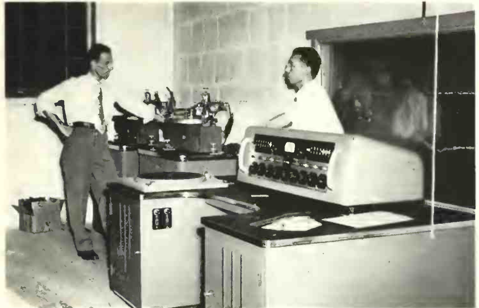
Disc recorders and control console being installed in Protestant Radio Center's headquarters, at Music Building of Agness Scott College, Decatur, Georgia.
