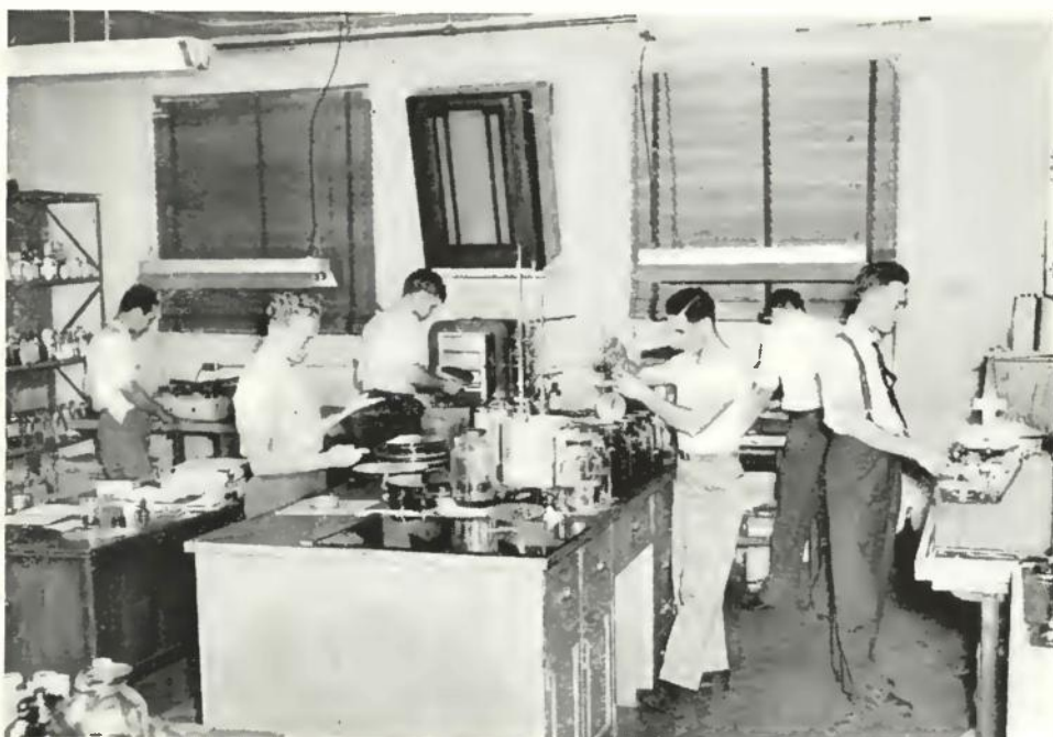
A section view of the new Audio Devices research laboratory in Stamford, Conn.
