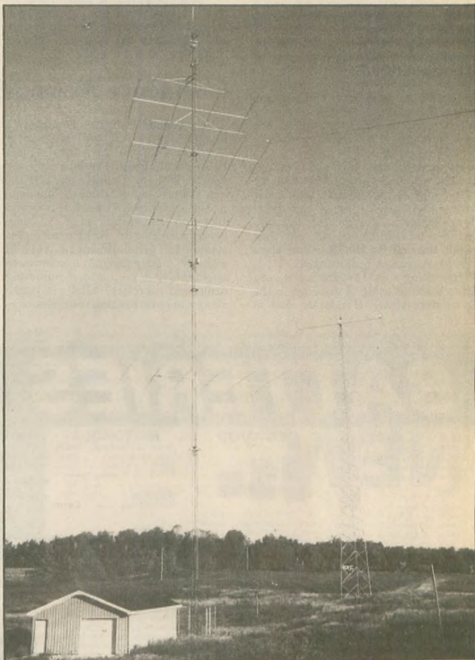
Rotating tower and 180 ft. self-supporting tower with 80M beam. Remote ham shack stands at the base of the 200 ft. tower.
