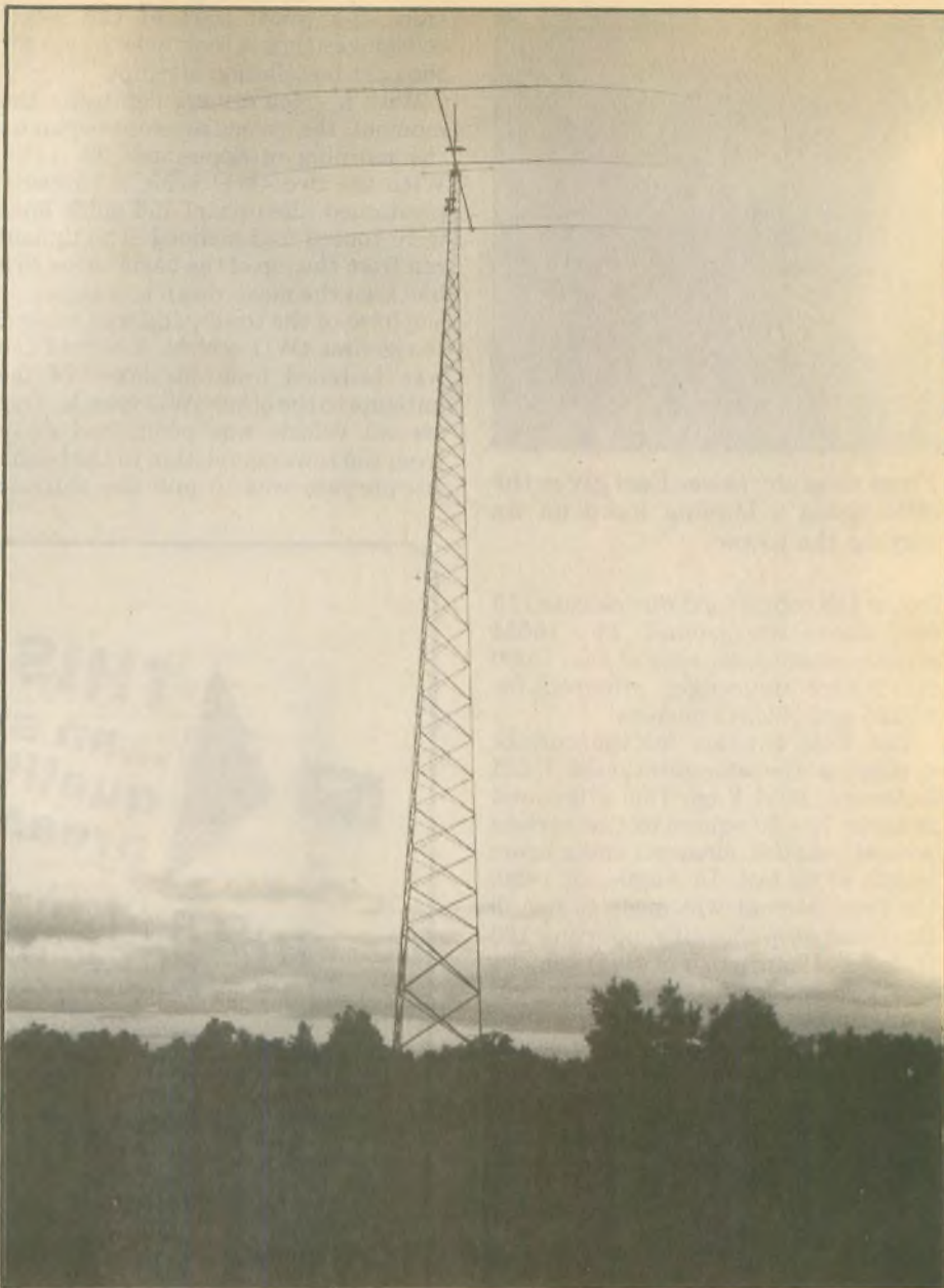
180 ft. tower with KLM 80M beam.
