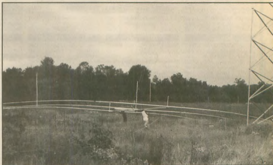
The 80M beam is gently lifted from the ground as it is prepared to be hauled to the top of the tower
