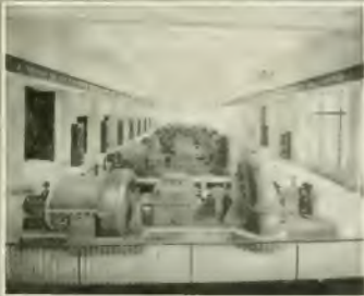
De Laval Municipal Water Works Installation
