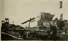
Tip-Works —In addition to the tipple or breaker (which houses the machinery for crushing, screening, washing and picking the coal), the tip-works in the modern coal mine includes power house, machine shop, sub-stations, warehouses, stables, powder houses and a complete company town for housing employees and their families.
