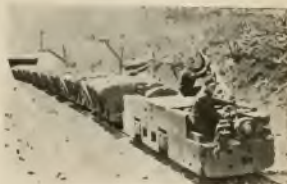
Hoisting Out the Coal —More than 20,000 locomotives—electric, steam and gasoline—operate on 200,000 miles of track in the coal-mining industry. About 50,000 miles of this trackage is electrified—equaling the combined length of the street and interurban railway mileage in this country.
