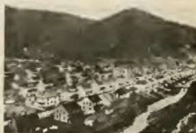
Coal Mine Village —The coal-mining industry houses between 7,500,000 and 1,000,000 people in villages like this. Lumber, roofings, paints, etc., are required in large quantities to build and to maintain these communities.
